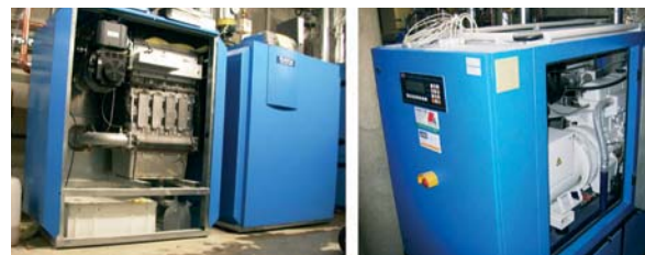
Two gas condensing boilers Combined heat and power unit
