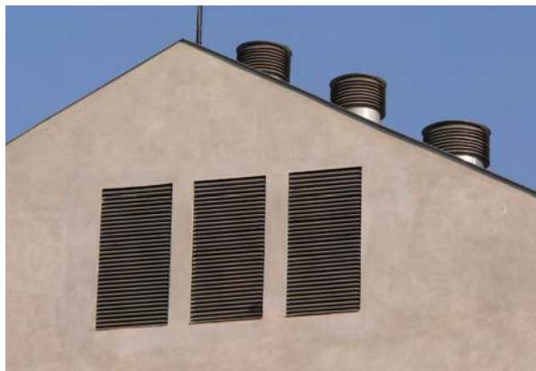
Air intakes and exhausts of the VRV air-conditioning system
