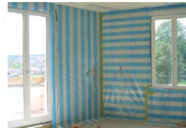
Internal insulation with vapour barrier
