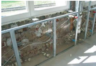
Aluminium frame for the internal insulation
