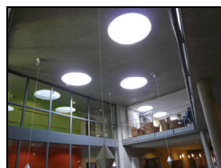
Roof skylights in the atrium
