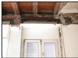
Interior view during construction
