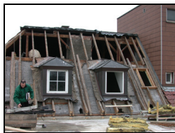
Renovation of the roof
