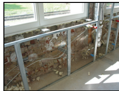
Aluminium frame for the internal insulation
