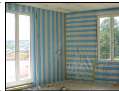
Internal insulation with vapour barrier
