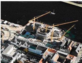
November 2005: top left: Library. top right: Opera House. bottom: Playhouse.
