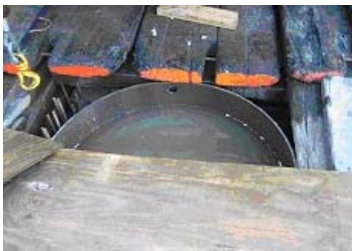
The top of the 120 m deep cold well.
