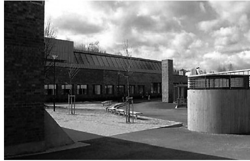
Pictures showing the main building before and after retrofit. Most visible features are the new daylight openings on the roof and new façades. The air inlet tower and a heat recovery unit (roof top) can be seen in the picture to the right. Architects for retrofitting: Hus Arkitekter AS. Photo left: B. Matusiak. Photo right: J. Rollan.
