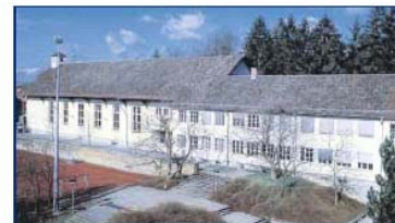
Figure 1: South view of the school building (building section 1 and 2)
