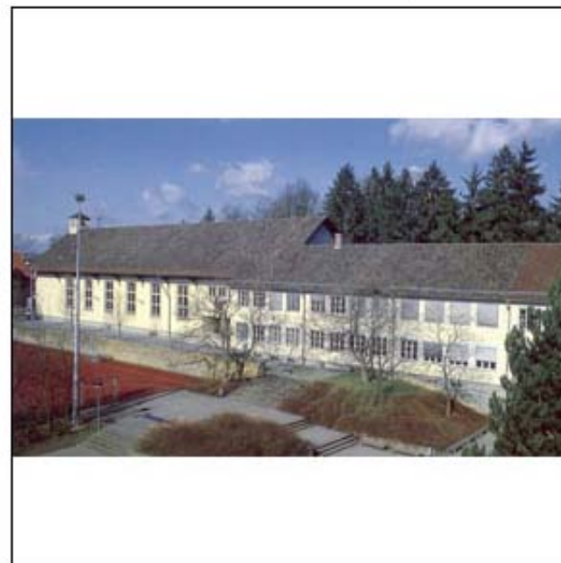
South view of the school building
