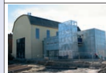
Cultural Centre Proevhallen
